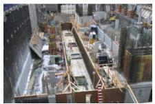
The design-build contractor for the new 12-story Alley 111 mixed-use high-rise in downtown Bellevue, Washington included a LEED-point eligible water retention vault to capture and store stormwater per the city's building code. This structure was constructed using a blind-side shotcrete method with Xypex Admix C-500 to ensure that it is watertight.
